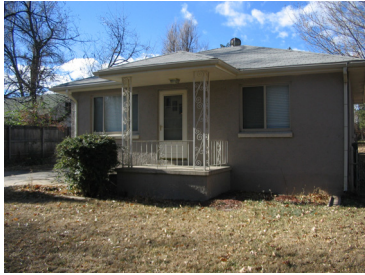
Existing Front Entry
